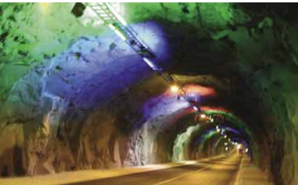
Tunnels are an important element in the infrastructure of the Faroes. The tunnel from Eysturoy to Borðoy established a road connection from the capital Tórshavn to the second-largest town, Klaksvík. It passes beneath the Leirvíksfjørður strait, reaching a depth of 150 metres below sea level. The colours come from a light installation by the artist Tróndur Patursson. Photo: Erik Christensen – Porkeri.
